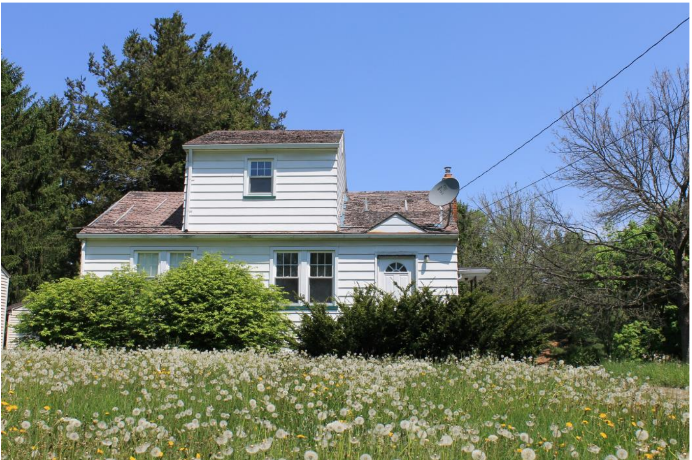
1924 Highlawn is a vacant property that is in need of significant repair
