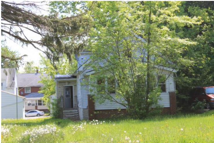
133 Matta Ave before demolition
