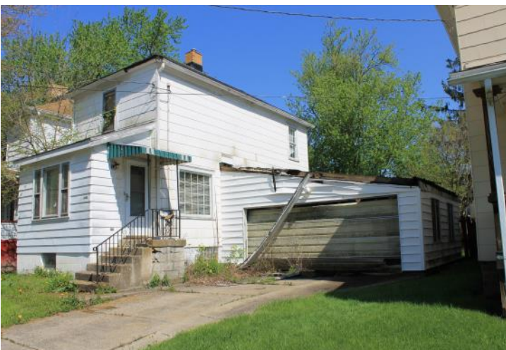
2442 Wilcox Street: DEMOLITION
