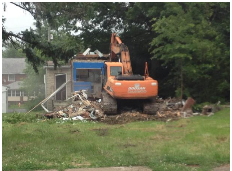
133 Matta Ave in the process of being demolished
