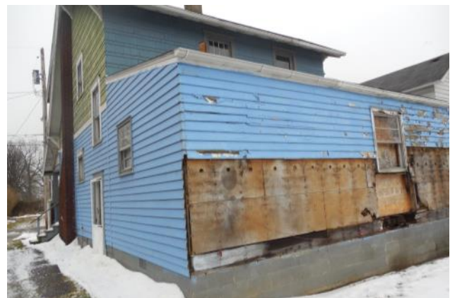
32 S. Richview Avenue: DEMOLITION
